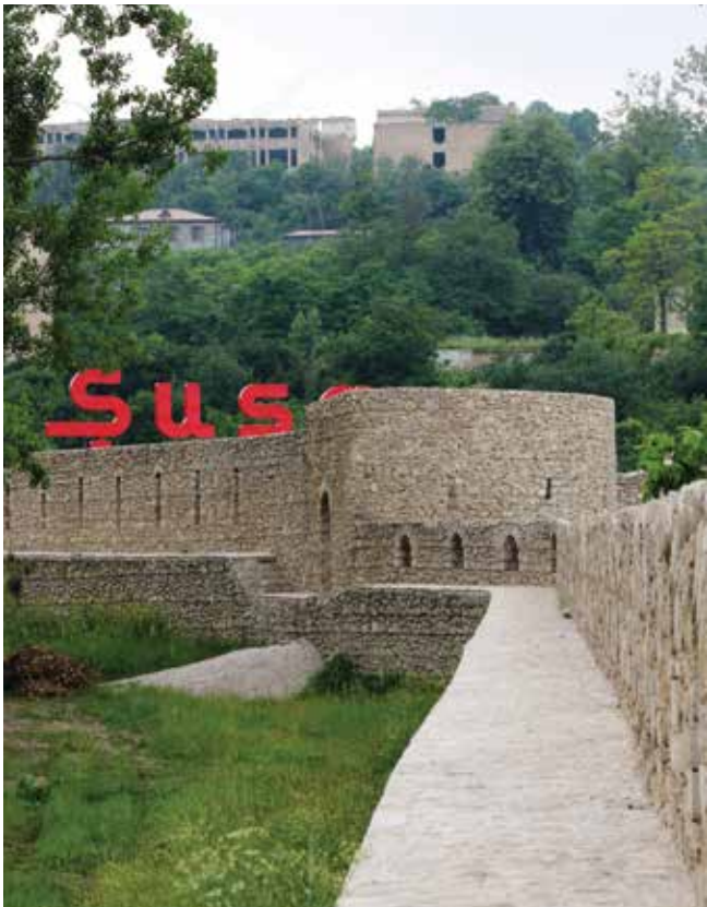
Fortress walls of the city of Shusha after restoration in 2023
