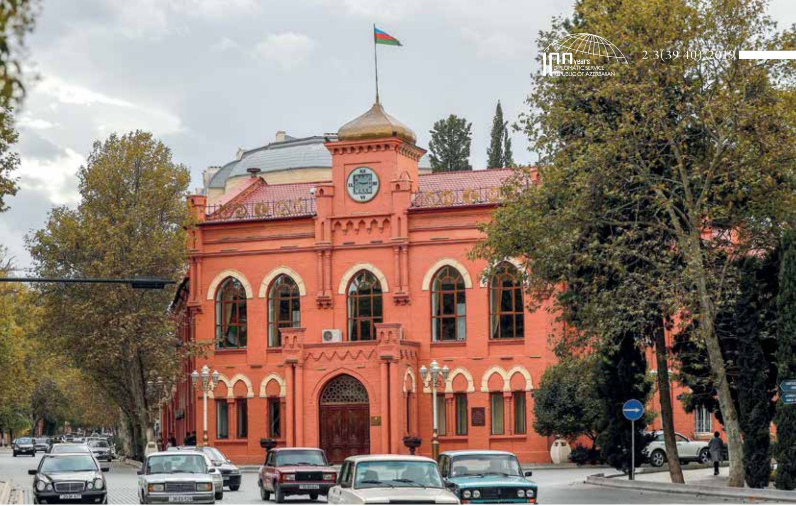
This building was the seat of government of the Azerbaijan Republic, including the Ministry of Foreign Affairs, in June-September 1918. Ganja, present-day photo
